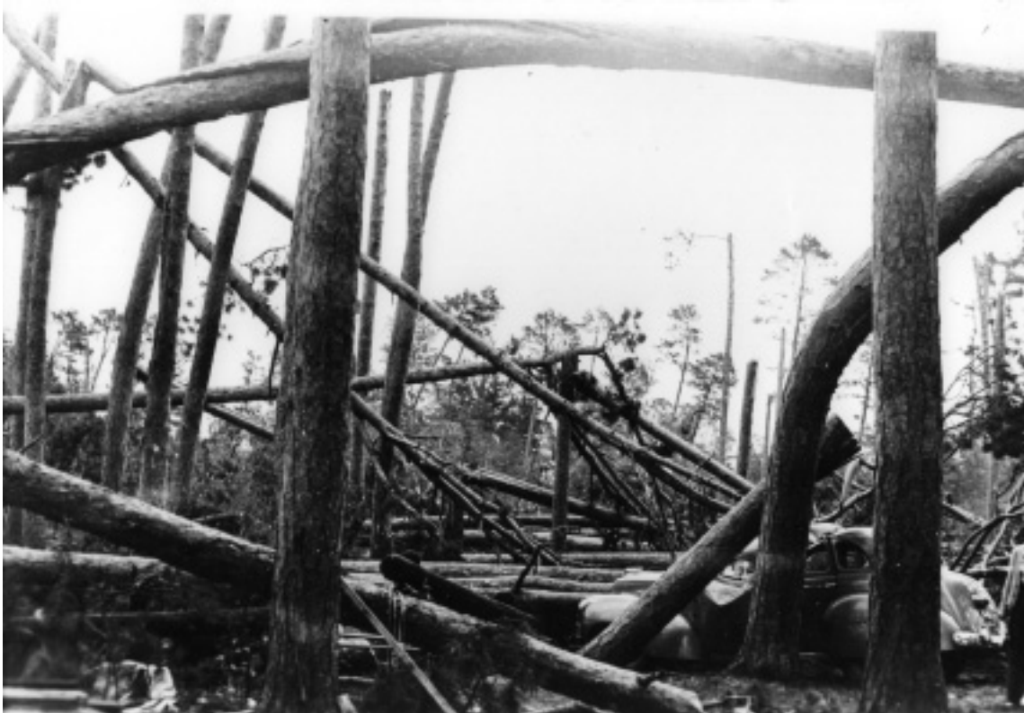
Storm Damage July 1940 at Norway Beach
